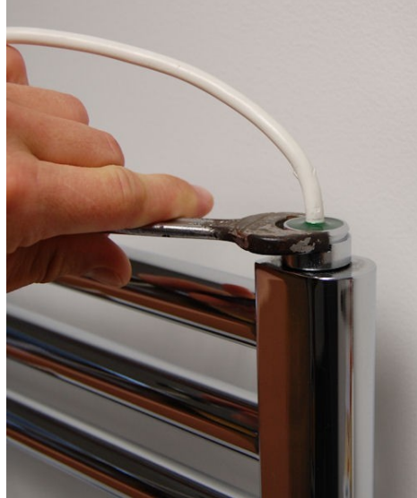
Nip to seal joint
