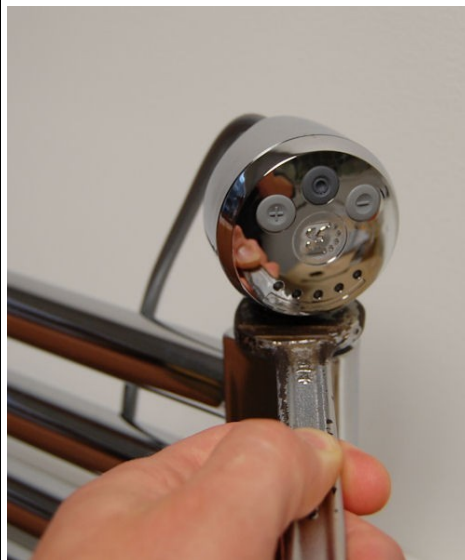
Align & seal using spanner
